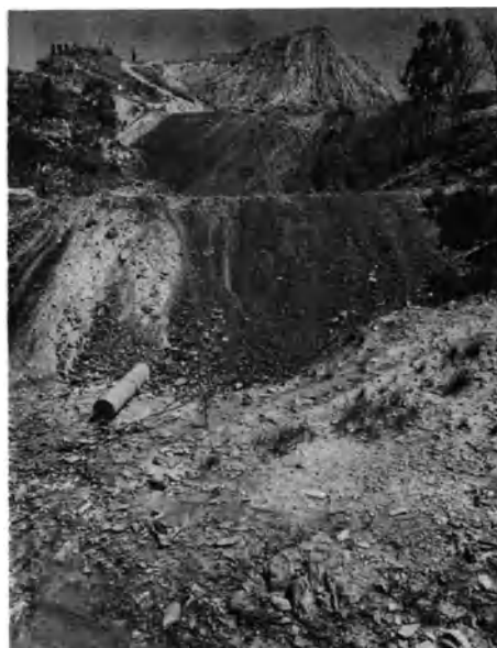
Figure 3: Drainage from the northern slimes and solids dumps passed through the pipe into the Molonglo River, causing it to be polluted and sterile for many kilometres.
